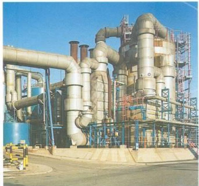
Figure 16.10 A Contact process plant used for making sulphuric acid
