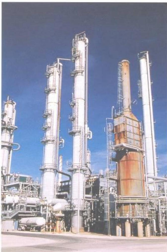
Figure 12.4 Fractional distillation of crude oil in a refinery.
