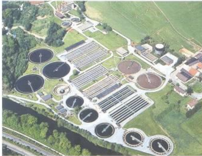
Figure 10.17 A water treatment works.
